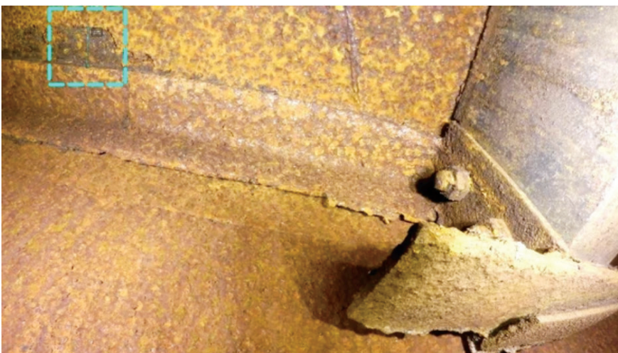
Corrosion Identified—Tank Joint Left Side
